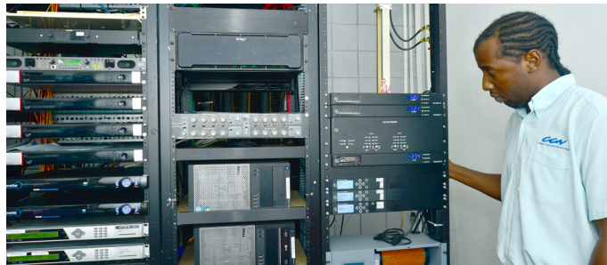
Brant Osborne , TECH Department, displaying the new digital station link implemented in 2013 which provides service for channel 6 at Gran Couva and channel 18 at Cumberland Hill.
