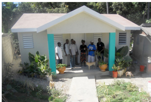
Here is an example of one of the 15 homes which were completed and handed over to families.
